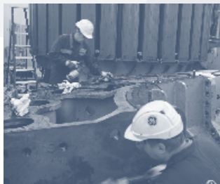
RENOVATION WORK IN KIERIKKI
