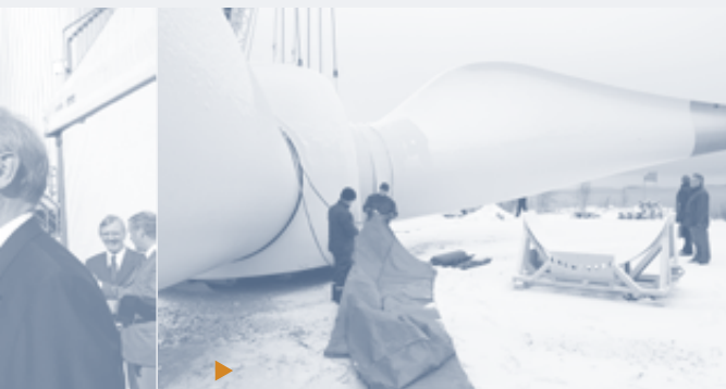
The largest wind power plant in Finland was erected at Vihreäsaari in Oulu in mid-November.
